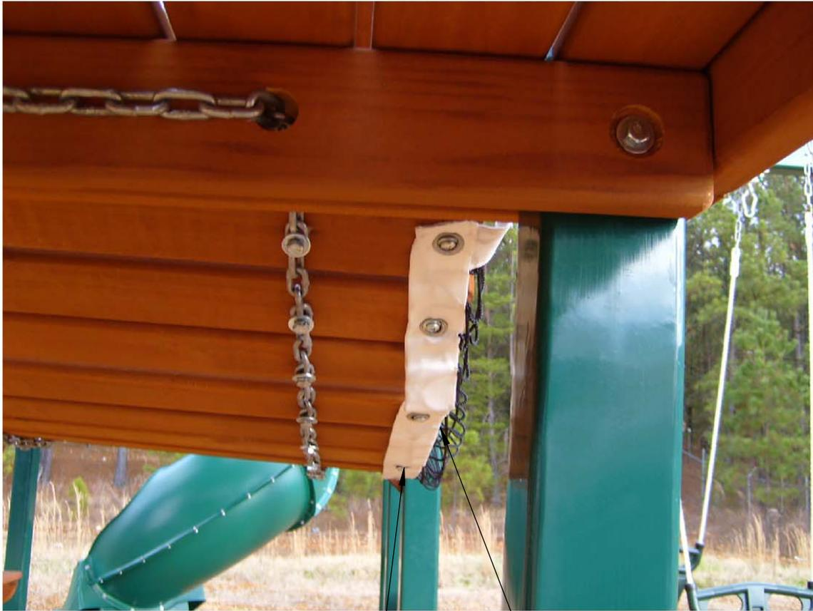
MARK THROUGH THE CENTER OF THE CENTER GROMMET ONTO THE MIDDLE DECK BOARD. DRILL A 1/8" X 1" DEEP HOLE AT THE MARK. PLACE A PAN HEAD SCREW THROUGH A WASHER AND INSTALL INTO THE HOLE. TRY TO CENTER THE WASHER ONTO THE GROMMET BEFORE TIGHTENING COMPLETELY.
